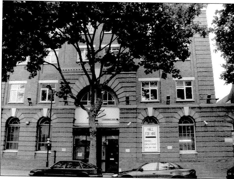
Figure 6: Live / Work at No.28 Lawrence Road
