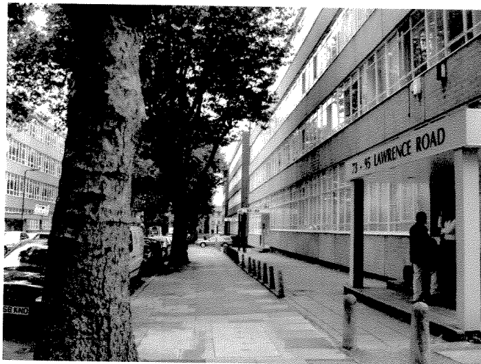
Figure 10: Street Frontage at Lawrence Road
